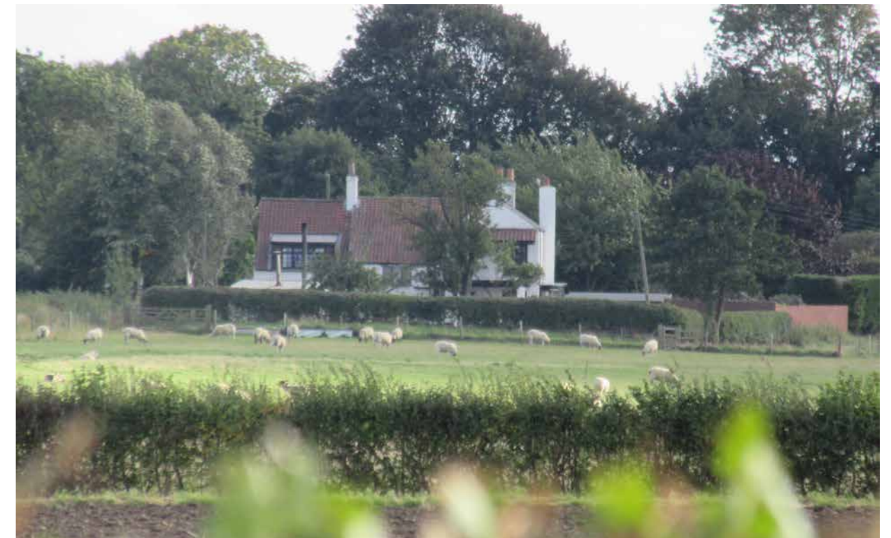
Fig 276: It is only from the public right of way leading from Corringham to Aisby that a reasonably open view can be gained towards Old Hall, the western parts of its grounds more porous and less wooded. From this view the general aesthetic of the building can be appreciated, with its white rendered facade and bright, steeply sloping pantile roof and collection of irregularly arranged chimney stacks.
