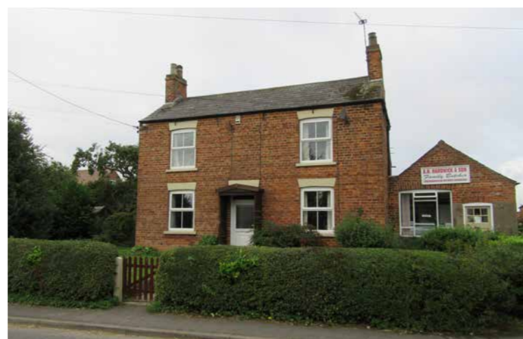
Fig 178: Built of red brick with a slate roof, No.7 Middle Street has a simple but pleasing vernacular aesthetic, with a well-proportioned, symmetrical facade. Adjoining the dwelling but setback from the principle elevation is single-storey block that previously accommodated the village butchers. Both structures can be seen on the 1885 map.
