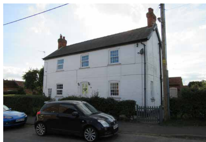
Fig 177: No.9 and 11 Middle Street has an L-shaped footprint, its east and south-facing elevations neatly marking the corner of Middle Street and Poplar Lane. Two storeys high, the converted farmhouse is built of brick, which is painted white, and has a slate pitched roof with red brick chimney stacks.
