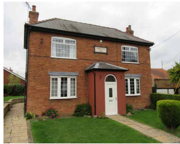
Fig 100: Built in 1929, as denoted in the inset stone inscription above the porch extension, Church View has a symmetrical 3-bay facade arrangement with slate hipped roof incorporating brick chimney stacks at either end.
