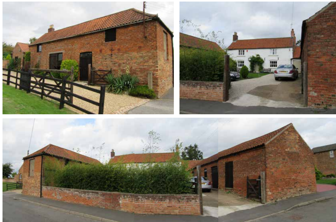
Fig 93-95: Mill House Farmhouse is an fine 18th century grouping with a simple courtyard arrangement. It comprises a centrally positioned farmhouse finished in colour-washed limestone with brick dressings, a single storey range of brick stables with segmental headed openings, and a brick barn. Pantiles dominate the roofscape and work in conjunction with the extensive red brick walling to unify the grouping.
