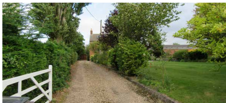
Fig 218 and 219: The farmhouse at Poplar Farm is tucked to the rear of its large front garden, with only its slate pitched roof and brick gable and chimneys viewable from the road. Nevertheless, with its classic vernacular form, handsome grounds and association with the neighbouring agricultural buildings, it stands as one of Poplar Lane's landmark dwellings.
