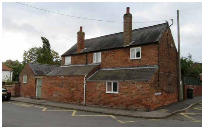
Fig 165: Now a private the residence, the original village schools was built in the early 1800s. Marking the southern-corner of Middle Street and East Lane, the building turns away from the street, with minimal fenestration across its red brick outward looking elevations. Two tall chimney stacks pierce the natural slate roof, adding visual interest to the upper extents of the building.
