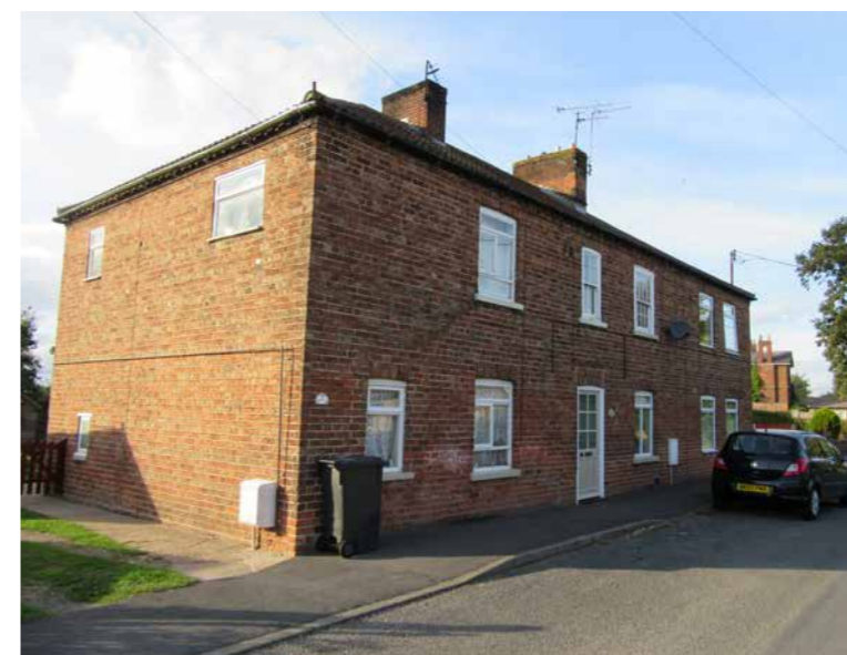
Fig 170: No. 39 and 41 Middle Street display a robust red brick form set below a hipped roof that hosts two broad chimney stacks along the ridge. Much of the original fenestration has been lost, though an 8-over8 timber framed vertical sliding sash remains at first floor level.
