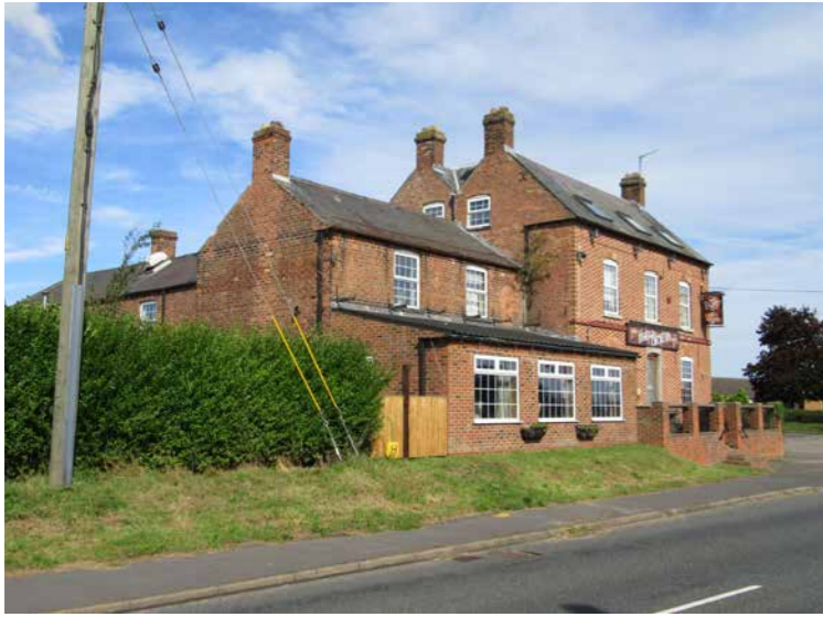
Fig 245: A local landmark and a stopping point for passing travellers since the 1800s, The Beckett Arms is one of Corringham's most distinct and locally iconic buildings. Though the focus of several alterations and expansion works, it is still possible to appreciate the buildings original red brick and slate roof form, with its unique M-shaped roof.
