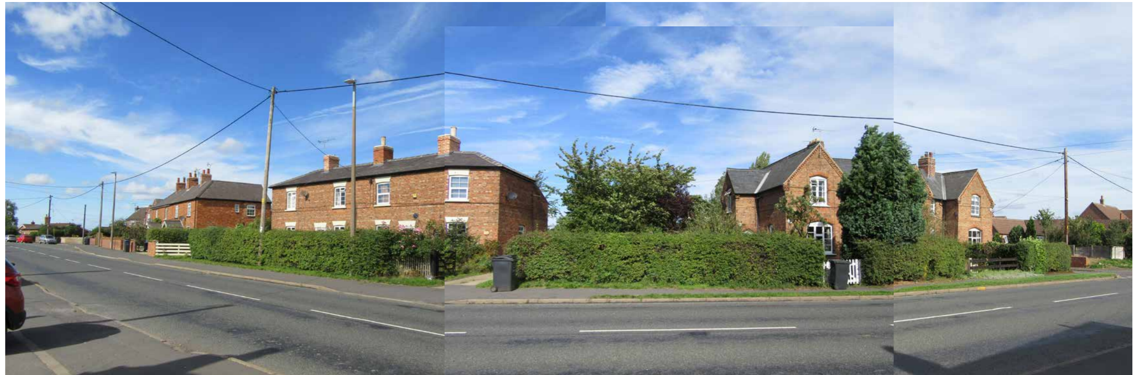
Fig 250: The sequence of semi-detached properties west of Poplar Lane represents one of the most unified and appealing historic groupings in Corringham.
