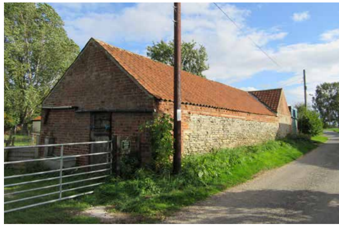
Fig 304: Still in use today, Thonock & Somerby Estates cattle boxes are made of what is locally called 'waterstone', a soft limestone with shells in it that is excavated from the earth below Aisby. This pale waterstone walling is complemented by the red brick and clay pantiles that characterise the buildings upper extents.
