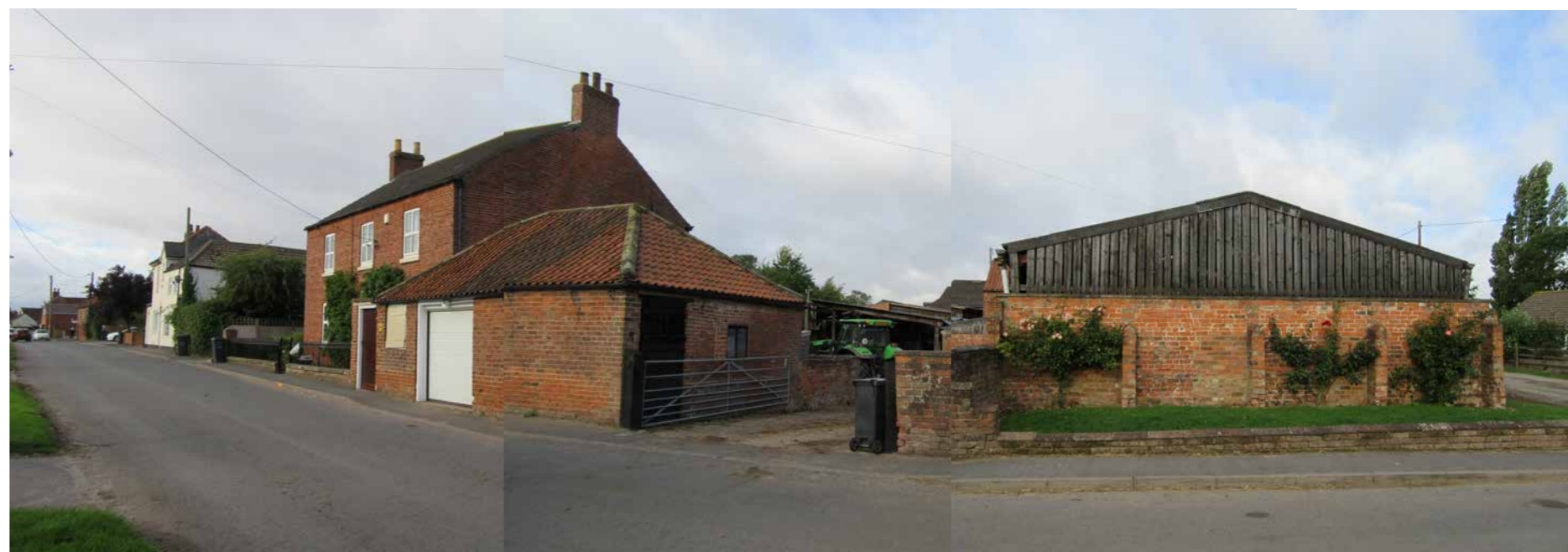
Fig 180: The red brick farmhouse and outbuildings at Red House Farm combines with the neighbouring white rendered property of No.27 Middle Street to form an extensive historic and handsome frontage along the roadside.
