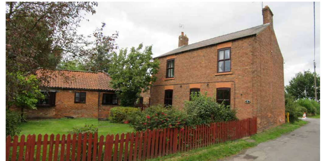
Fig 101: Positioned at the far northern end of Church Lane, Swallow Cottage is a traditional farmstead built entirely of red brick. The two-storey farmhouse has a slate roof with chimneys emerging from either gable end, whilst the single-storey outbuilding is roofed with pantiles.
