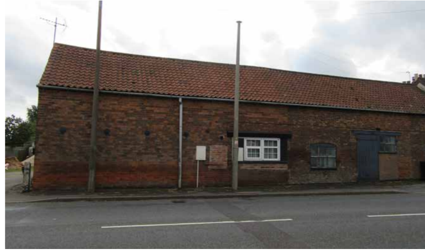
Fig 246: The former Thonock & Somerby estate workshop building presents a long, largely blank frontage along the southern edge of High Street. The right-hand side of the facade includes original fenestration and the plank entrance door.
