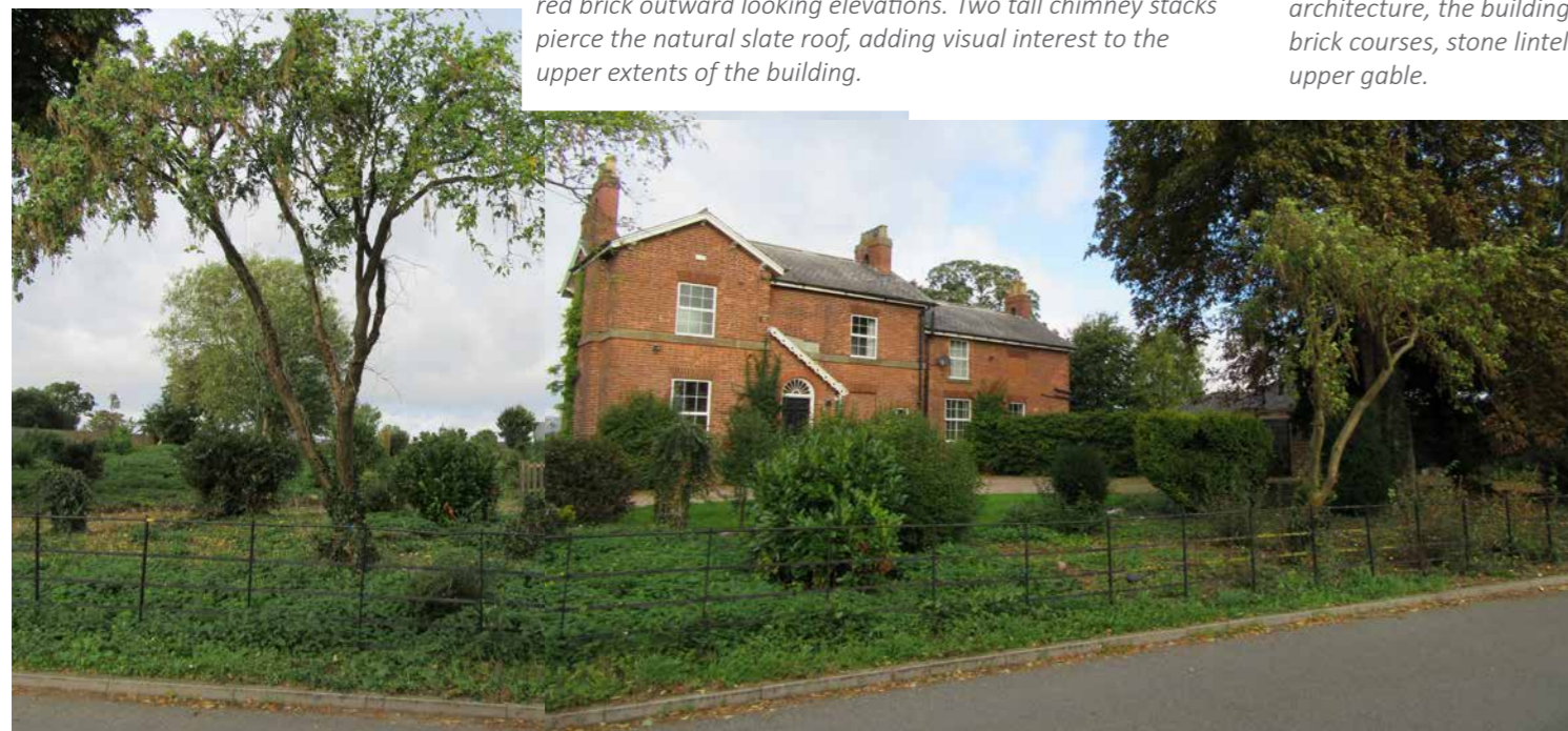
Fig 169: The former vicarage stands in mature grounds along Middle Street. One of the village's key landmark buildings, the vicarage is a grand residence built of red brick with slate roofs. Notable details include a mono-pitched porch with decorative timber eaves, a stone string course above ground-floor level, fanlight above the entrance door, twelve light sliding sash windows, and tall brick chimney stacks with distinct arched voids.
