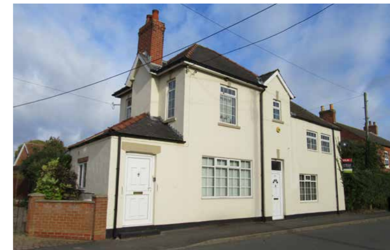
Fig 168: Formally hosting the village post office and grocery, No.27 Middle Street is today a private residence. In addition to this change of use, in recent times the building's red brick form has also been rendered and its windows and doors replaced. However, these changes aside, the building remains relatively true to its 19th century form.
