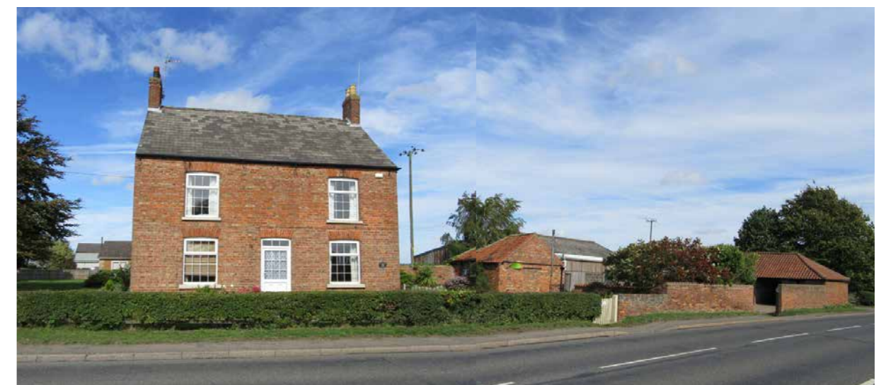
Fig 244: Corner Farm is a key gateway building stood prominently at the southern entrance to Middle Street. One of Corringham's best preserved farmhouses, the dwelling has a locally distinct red brick and slate fabric, with the introduction of uPVC windows being the only notable external alteration carried out since its construction. Sharing a setting with the farmhouse are a pair of traditional agricultural outbuildings, both of red brick with pantile roofs.
