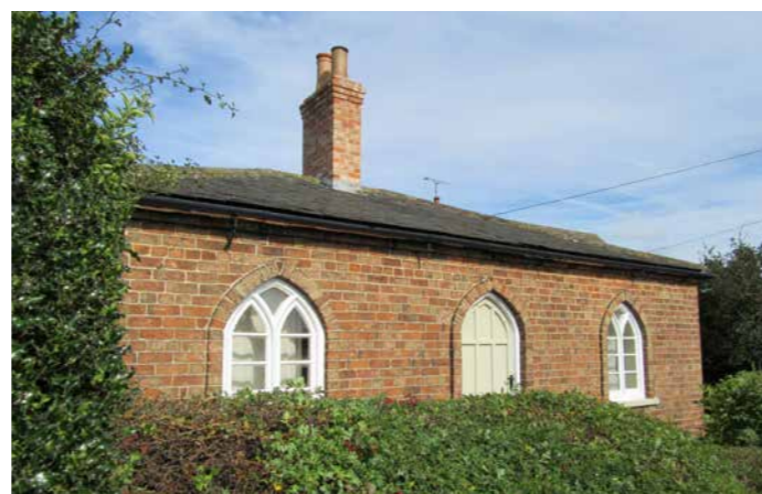
Fig 243: The A631 was originally the Towland to Hainton toll road, and this former status is celebrated by the still standing toll house at No.1 High Street. A Grade II listed building, the toll house dates from the early 1800s and is a charming and eye-catching prescience along High Street. Its 3-bay front contains a central planked door flanked by 2 light glazing bar casements, and is topped by a hipped slate roof and central brick stack.
