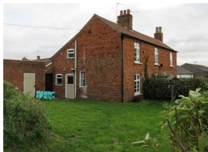
Fig 176: Originally a farmstead, but now a pair of semi-detached dwellings, No.26 and 28 Middle Street stand set back from Middle Street and perpendicular to the road, the buildings distinct side-profile, with cat-slide roof, facing towards the street.
