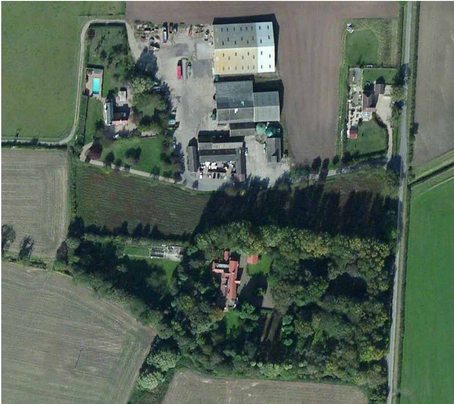
Fig 281: The aerial view of Old Hall and Hall Farm highlights the contrasting character of the two sites, with Old Hall set within particularly mature and densely wooded grounds, and Hall Farm much more exposed and open to the wider landscape.
