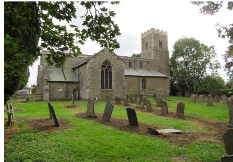
Fig 71: Constructed of coursed limestone rubble with ashlar dressing and lead roofing, St Laurence's is Corringham's most iconic and longest-standing building, parts of which date from as early as the 11th century.
