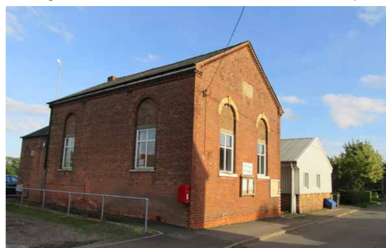
Fig 179: Corringham's village hall is a community hub and one of the settlements most distinct and instantly recognisable historic buildings. Originally the settlement's Wesleyan Methodist Chapel, as hinted by the 'Wesley' in the slightly eroded stone plaque on the upper gable, the building was converted into the village hall in the 1960s.
